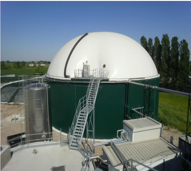
Full scale AD plant with enzyme treatment
