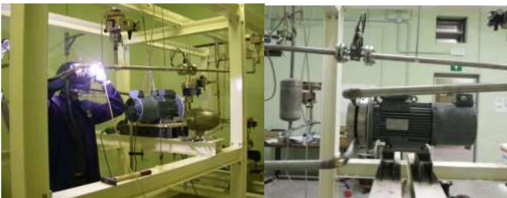
Figure 4 - installation of the pump and final configuration
